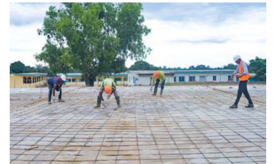
Construction of sports ground at Mandji's High School.
