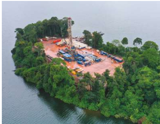
Compact pad and minimal civil infrastructures at Ngongui-3 during E&A activities.
